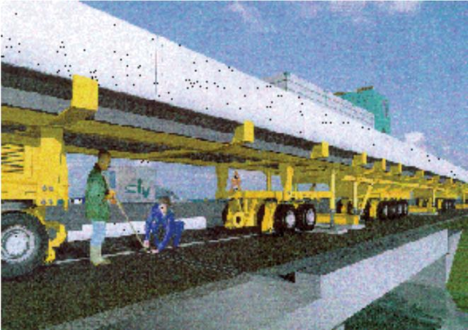
Other smart solutions like temporary 'bridges' are used to roof over maintenance work, thus relieving congestion, reducing the need for diversions and creating safe conditions for the workers<sup>34</sup>.
