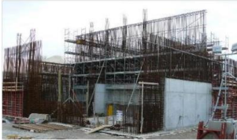
Figure 31: DMC3 and DTC3 construction
