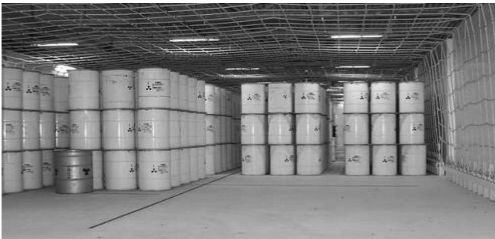
Figure 4: Caorso NPP – ERSBA 2 storage facility
