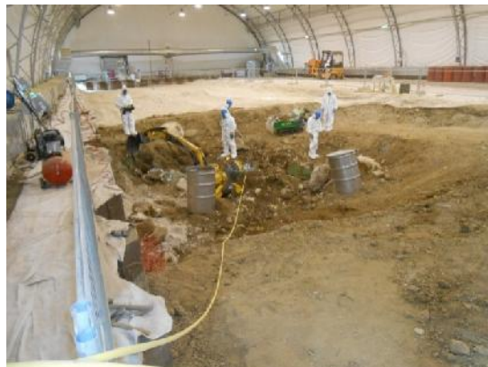
Figure 25: Trenches remediation activities
