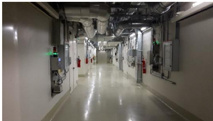
Fig. 42 New OPEC-2 store completed and waiting for operating permit
