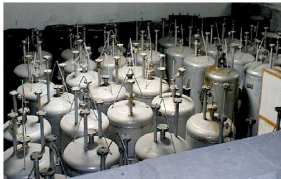
Figure 5: TRINO NPP – Resins from past operation stored in the site
