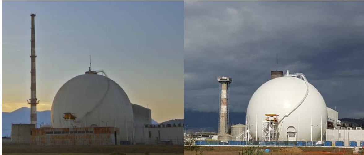
Figure 15: The chimney of the Garigliano NPP under dismantling
