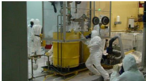
Figure 33: Cleaning of the bottom pool
