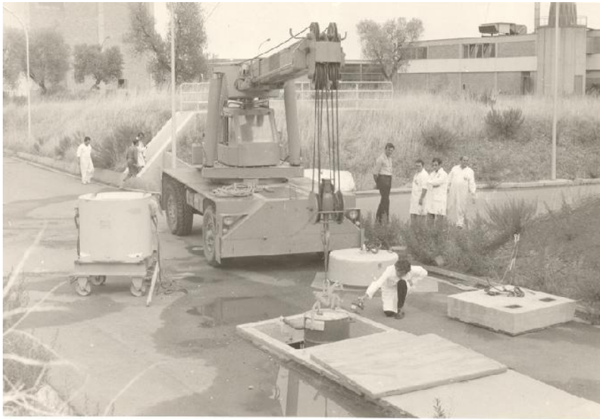
Figure 14: Historical picture of burial of radioactive waste in pits at the ITREC facility in the years '70s.
