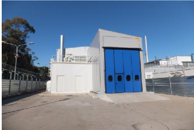
Fig. 40 Waste A&B dismantling facility at OPEC-1 plant
