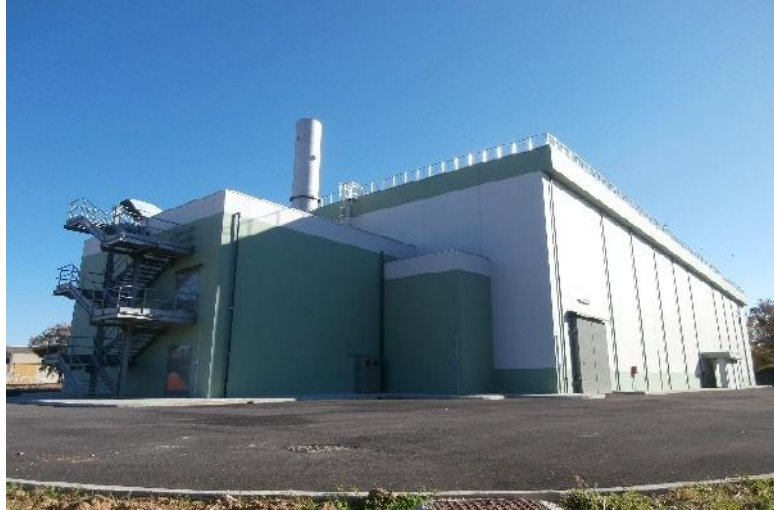
Figure 7: Latina NPP – New storage building
