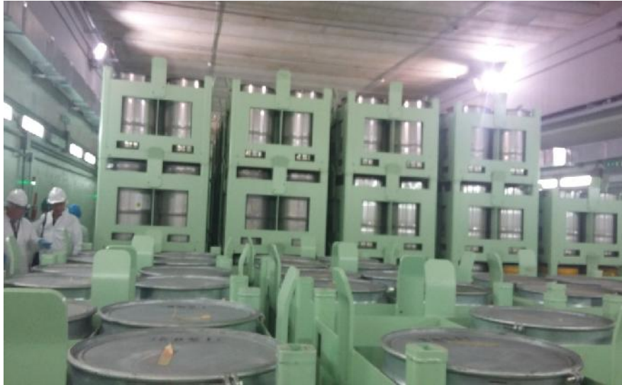
Figure 6: Garigliano NPP – D1 storage facility
