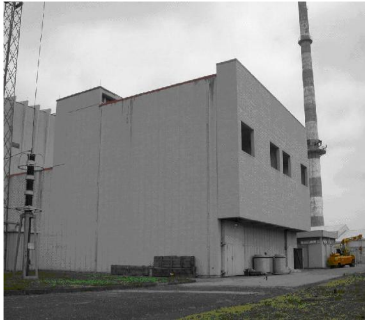
Figure 22: Storage facility "ex Diesel"
