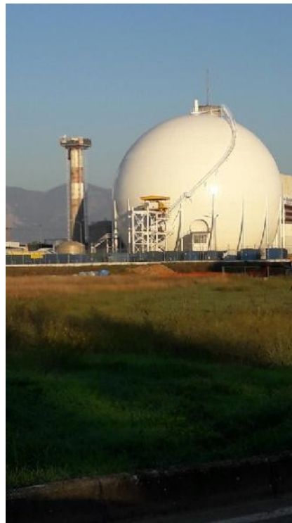
Figure 23: Garigliano NPP plant stack
