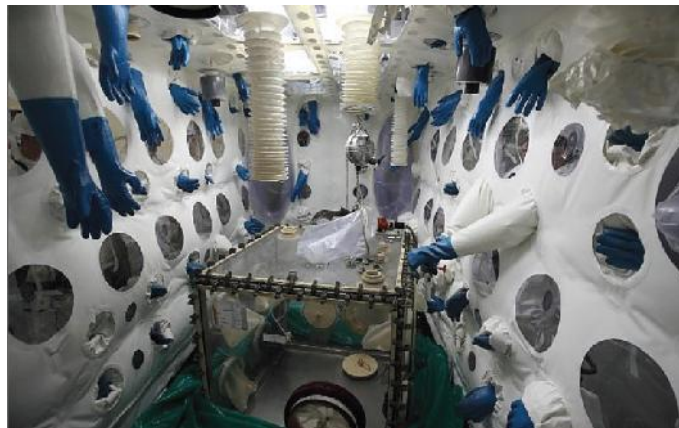
Fig. 41 Glove box dismantling at Plutonium plant
