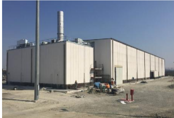
Figure 28: Waste storage facility "D2"
