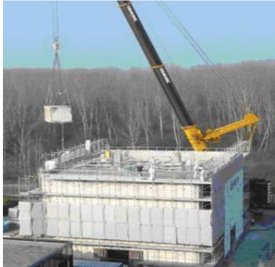
Figure 18: Caorso NPP - Off-gas building dismantling
