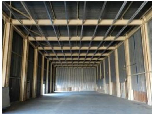
Figure 39: Refurbishing activities of building B106
