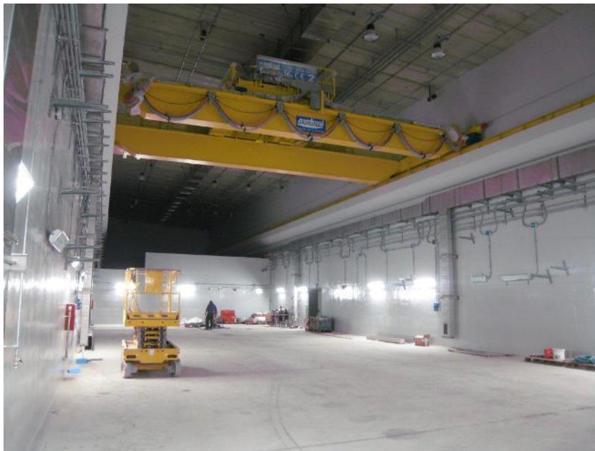
Figure 8: EUREX D2 storage facility
