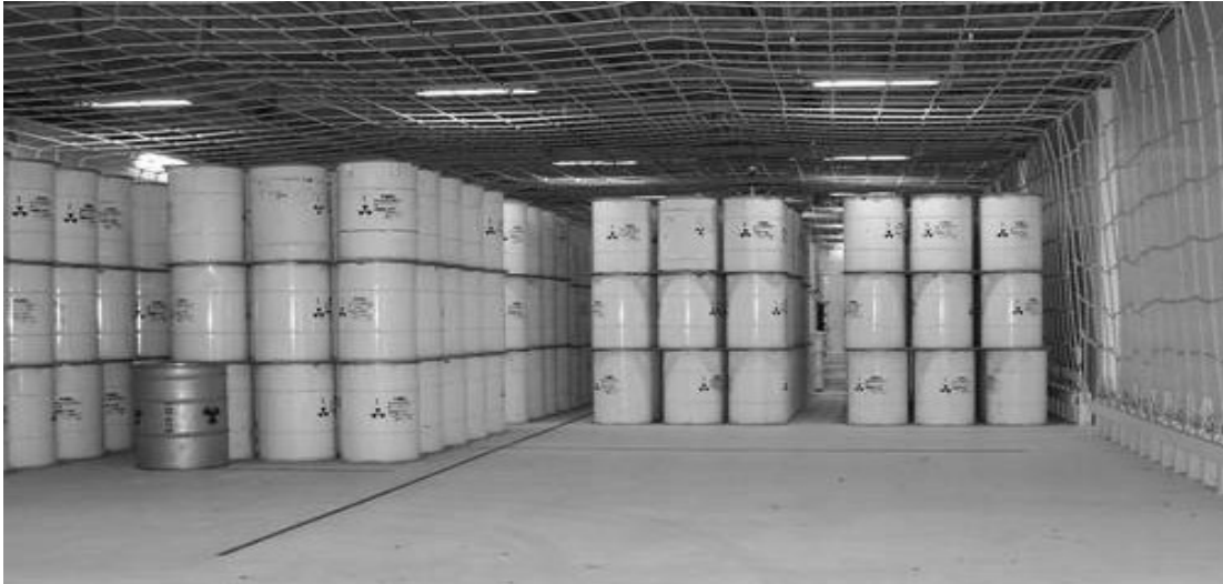
Figure 3: Caorso NPP – ERSBA 2 storage facility
