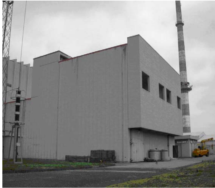
Building storage ex-diesel
