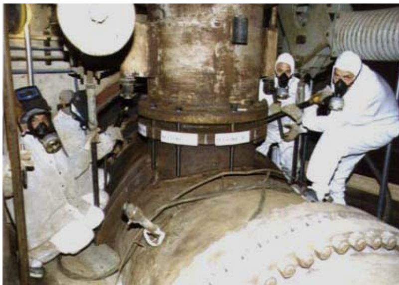
Figure 5: Latina NPP – Preliminary dismantling activity of the primary circuit
