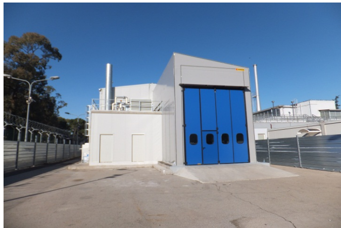
Figure 1 – Waste A&B dismantling facility at OPEC-1 plant
