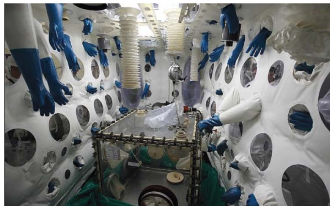
Figure 2 – Glove box dismantling at Plutonium plant
