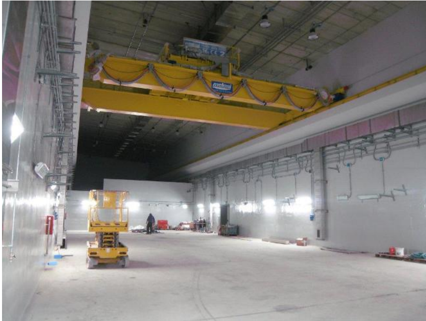
Figure 6: On-going construction of D2 storage facilities
