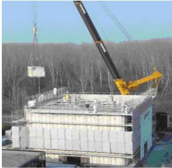
Caorso - Off-gas building dismantling
