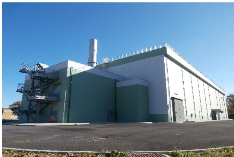
Latina new storage building
