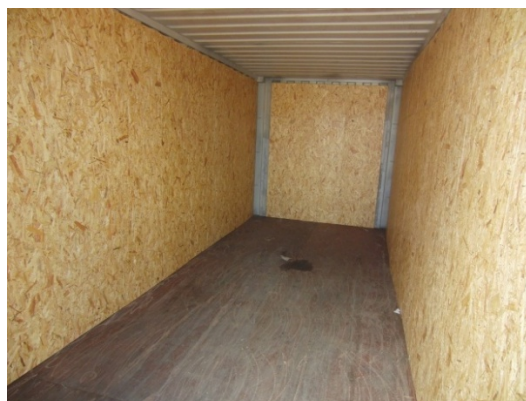
Figure 7.53 Lining a 40-foot container with chipboard panels
