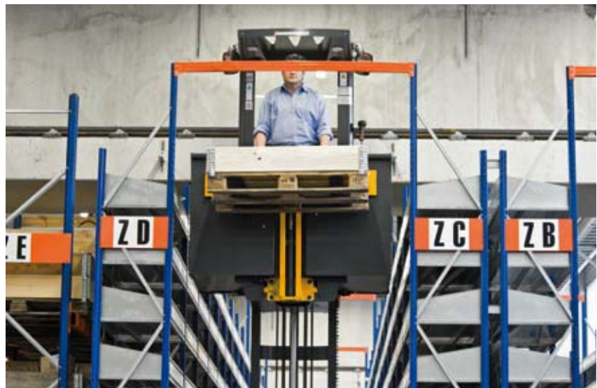
Lift and travel cut-out
