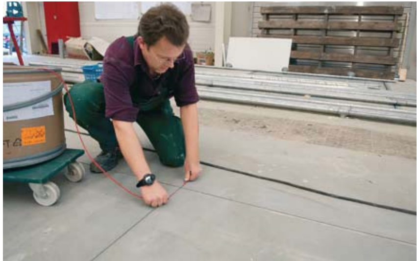
Inserting the cable
