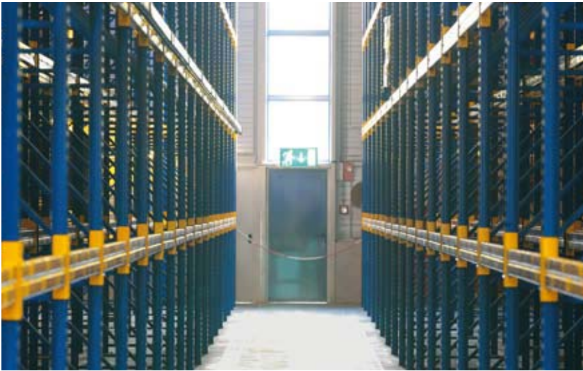
Escape door at the end of the working aisle
