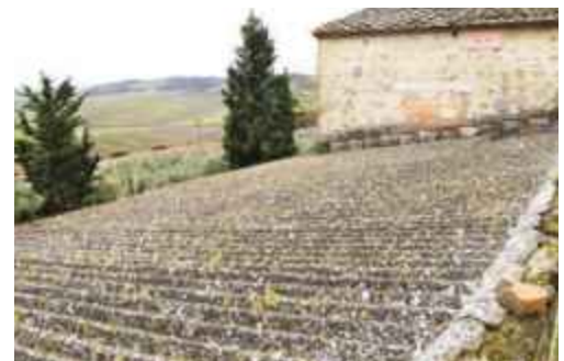
Roofs in good condition can remain in place
