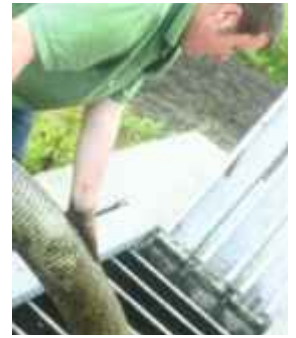
Safe removal of slurry
