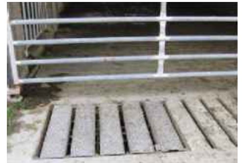
Replace covers at the end of work
