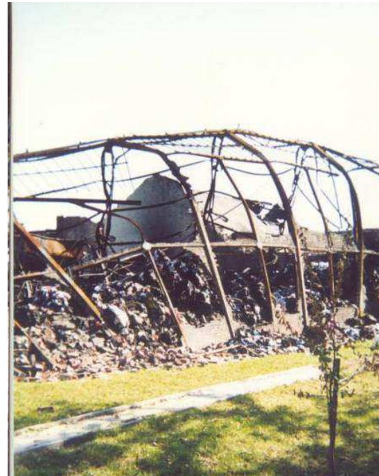
Figure 2-1 Prestressed concrete structure fallen OUTSIDE (above) and steel structure fallen INSIDE (right)
