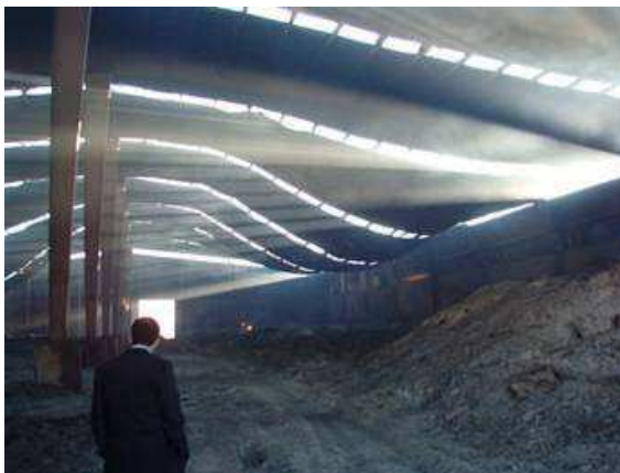
Figure 2-2 After fire, partial collapse
