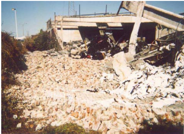
Figure 2-1 Prestressed concrete structure fallen OUTSIDE (above) and steel structure fallen INSIDE (right)
