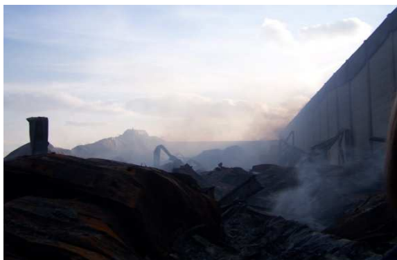
c) Firewall not damaged by the fire
