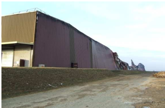
a) Damaged building after the fire
