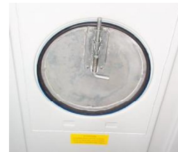
Figure 12.2-2: Roof hatch internal lock
