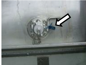
Figure 12.2-7: Top valve seal
