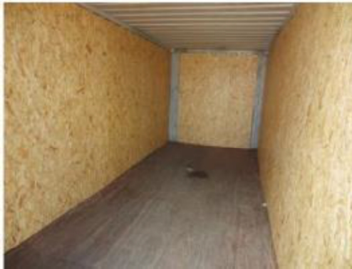
Figure 10-78 Lining a 40 ft container with chipboard
