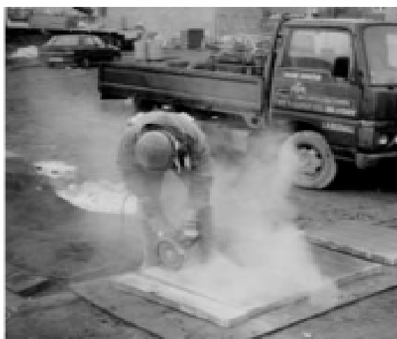
(a) Figure 3 Slab cutting using LEV: (a) without control; (b) with control
