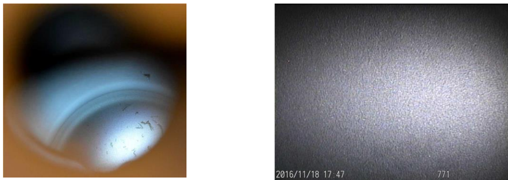
Figure 17 Internal views of cylinder L89.2
