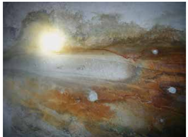
Figure 3. Local corrosion on a stainless steel tank surface.
