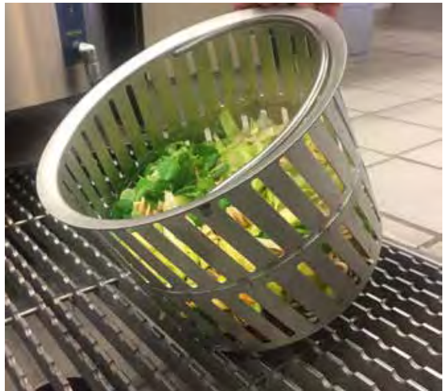
Figure 5. A 7-litre filter basket that is filled halfway allows full flow. A channel filter can hold back waste before it enters the channel.
