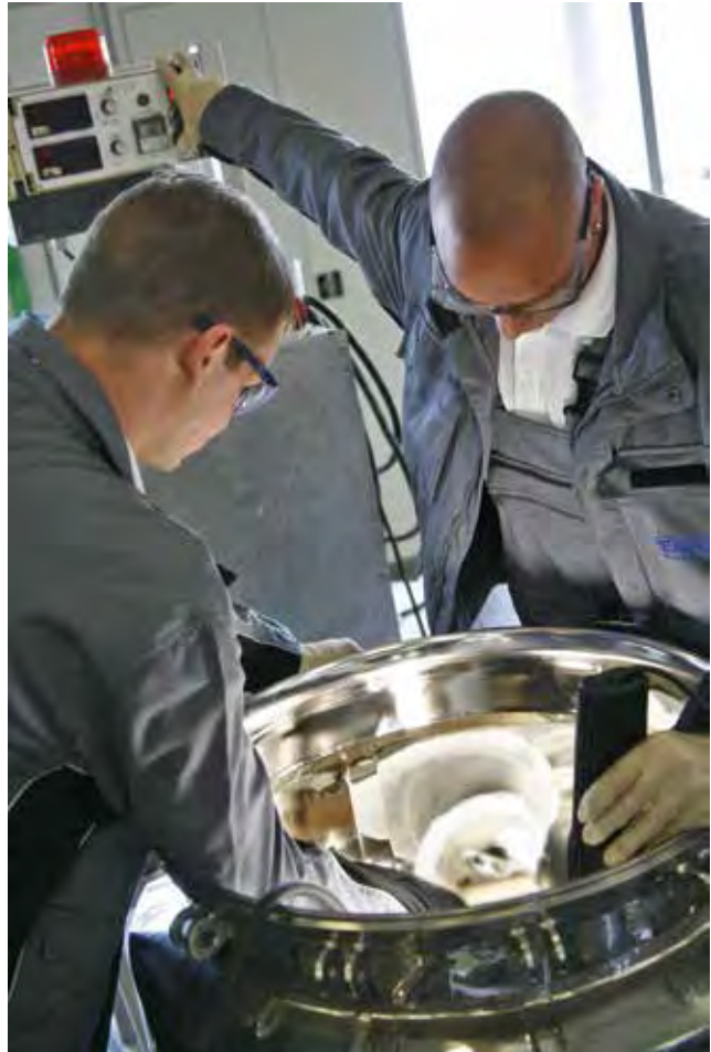
Figure 5. Local refurbishment by electropolishing on-site.
