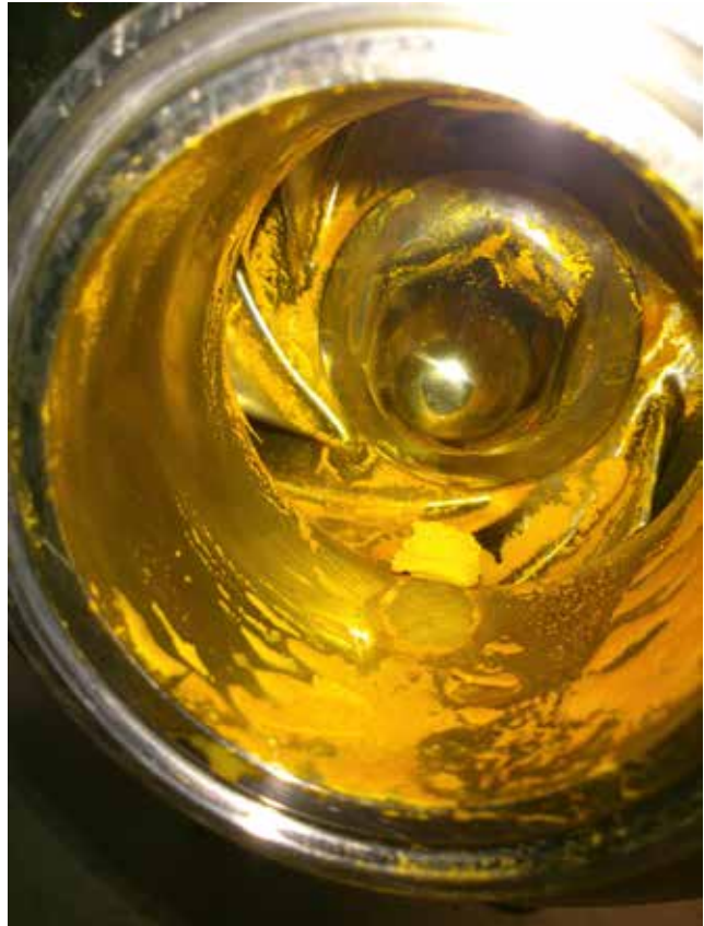
Figure 3. Assessing a centrifugal pump during trials at AINIA
