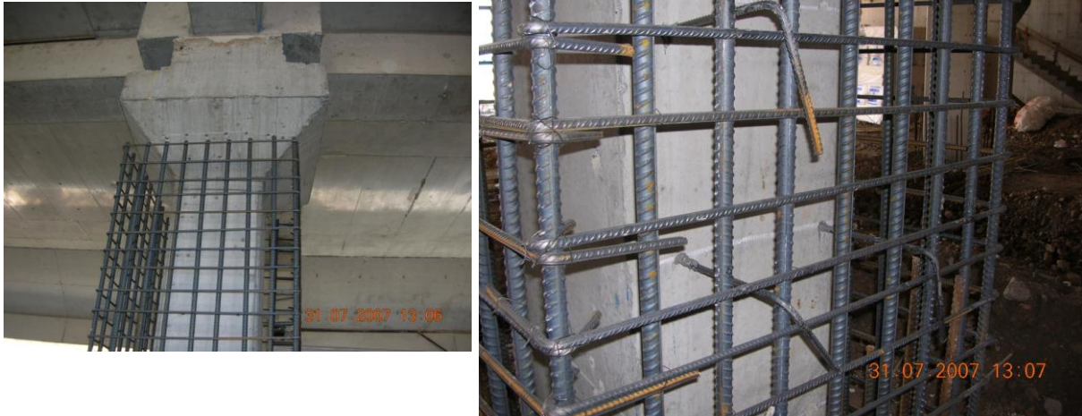
Figure 9.2 Application of RC Jacketing to a column
