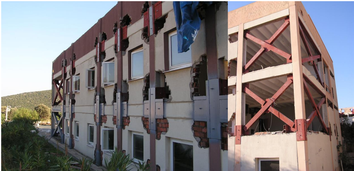
Figure 9.7 Retrofit using steel bracing
