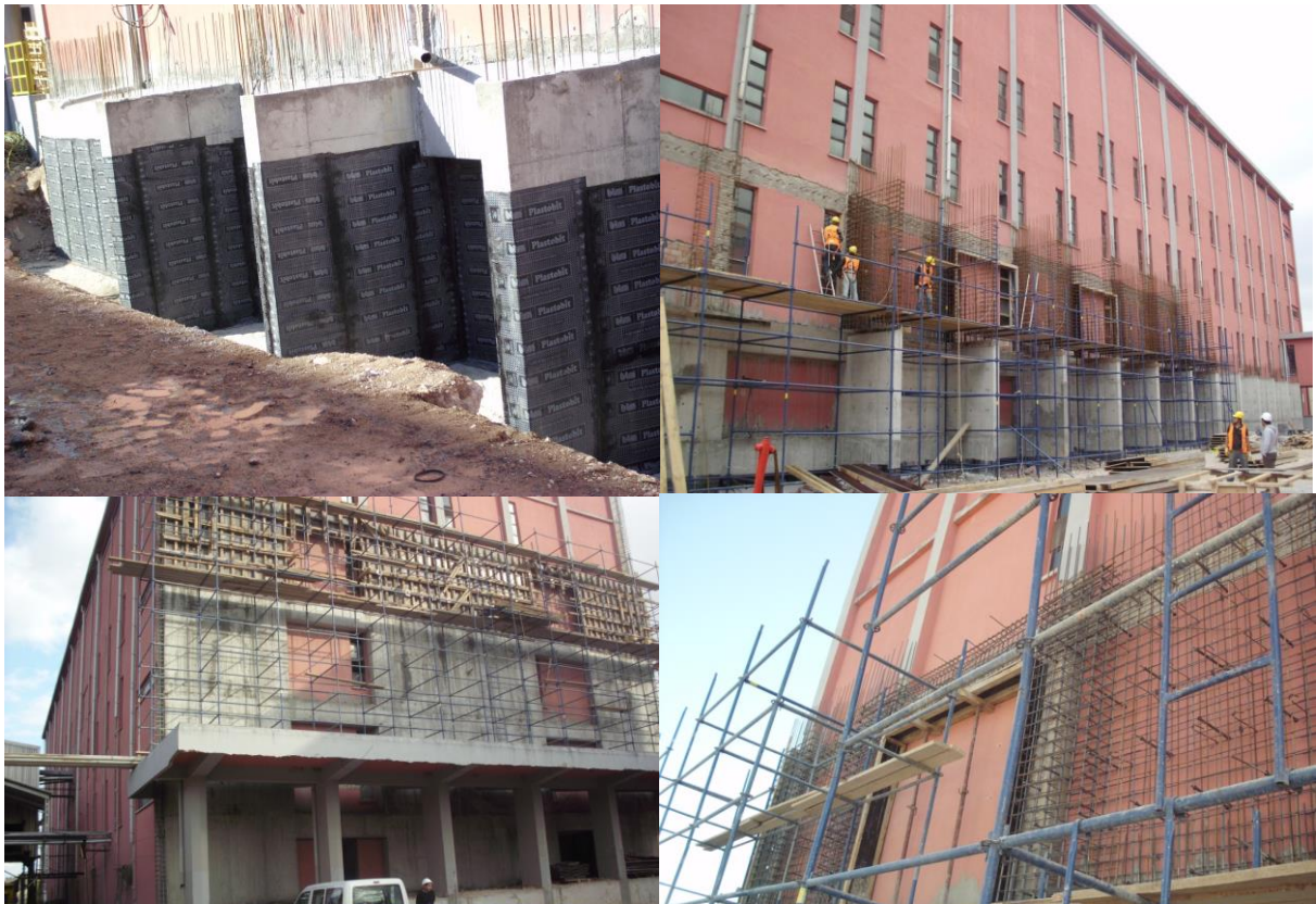
Figure 9.9 Various stages of construction
