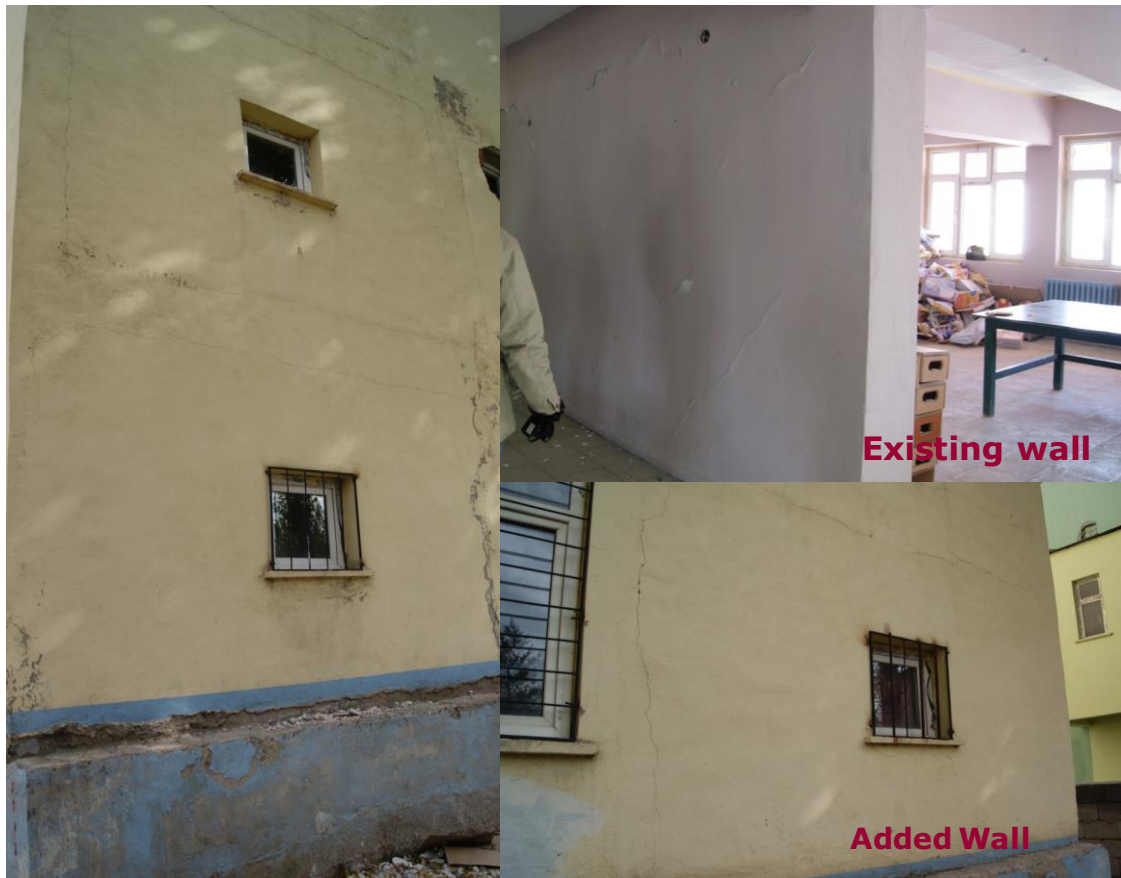
Figure 9.11 Performance after 2011 Van Earthquake
