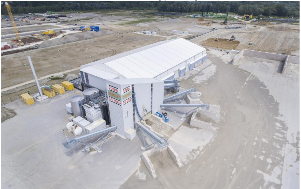
Figure 2: Aerial view of the soil washing plant (front), sludge treatment facility (left hand side) and the reception hall (in the back). Copyright: ARGE AUDI IN-Campus GbR.
