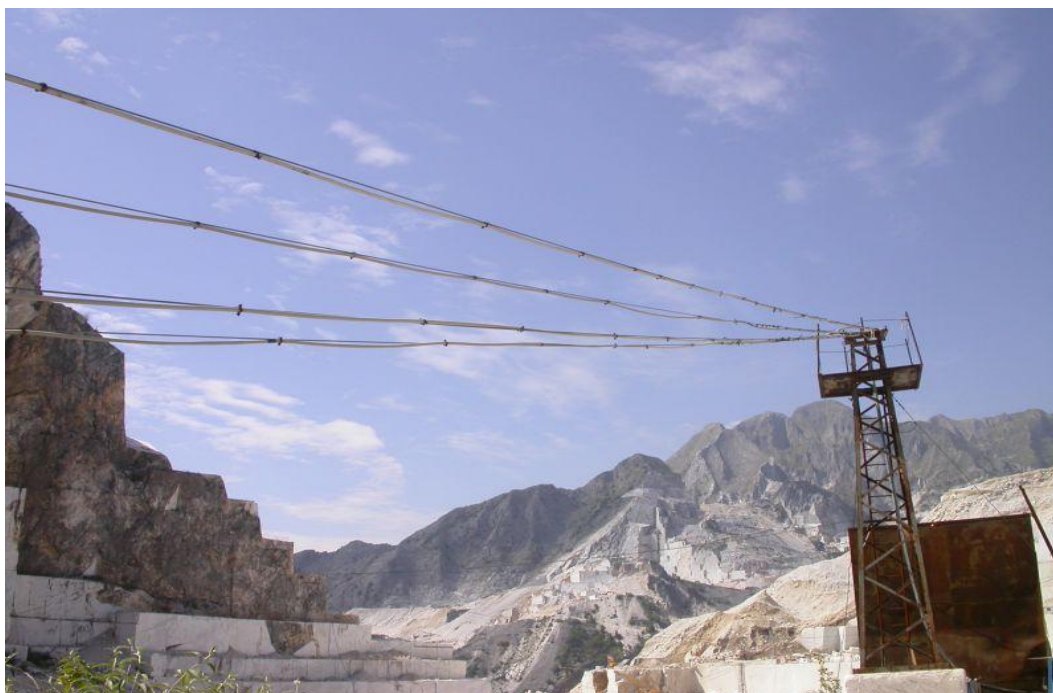
Foto V.1.1 – Linee aeree in cavo
