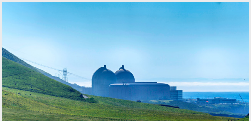
Diablo Canyon nuclear power plant, USA.
