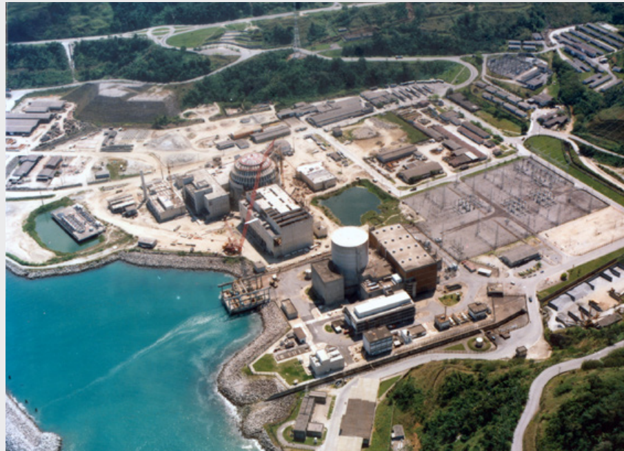
Angra nuclear power plant under construction, Brazil.
