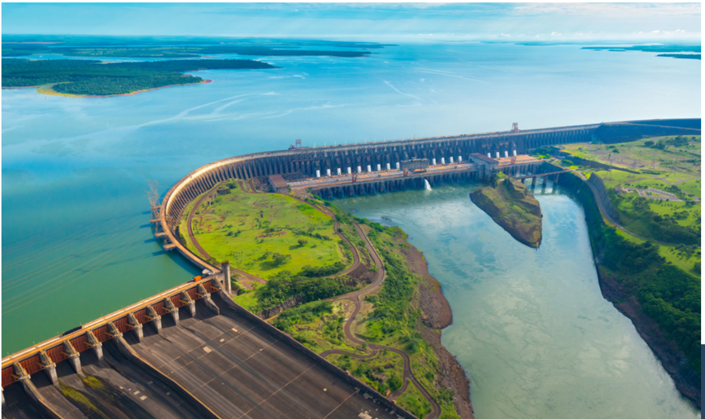
Itaipu Dam located between Brazil and Paraguay.
