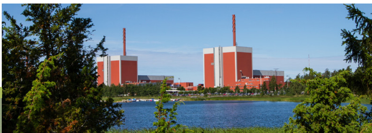
Olkiluoto nuclear power plant, Finland.
