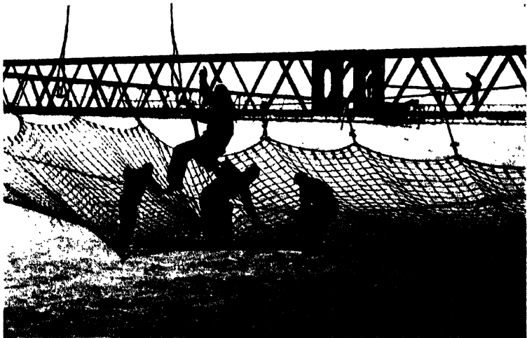
FIG. 86.—Huge life nets for the protection of workmen on the San Francisco-Oakland Bridge. (Courtesy of Safety Engineering-Acme Newspictures, Inc.)
