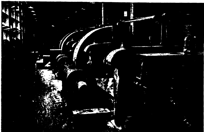
FIG. 108.—Rubber mills with inclosed gears. The ruggedness and simplicity of complete gear inclosures as compared with less perfect protection are well portrayed here.
