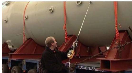
FIG. 5. Arrival inspection of a large heat exchanger.
