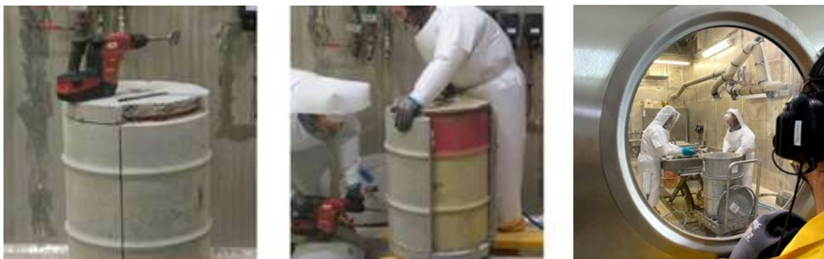
FIG. 6. Removal of the pre-cut concrete liner to gain access to the inner drum.
