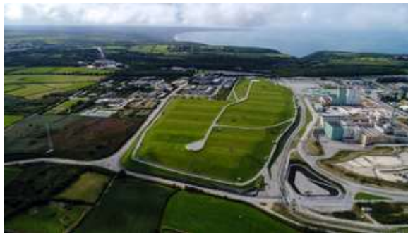
FIG. 4. Aerial view of the CSM. Courtesy of Andra
