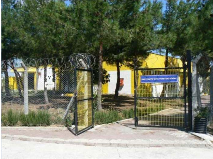
FIG. 2. Radioactive waste processing and storage facility.
