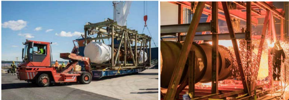
FIG. 10. Transport of Top Gas duct (left) and segmentation of gantry (right).
