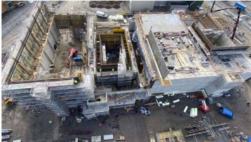
FIG. 4. On-going construction of Posiva's encapsulation plant. Courtesy Posiva Oy.
