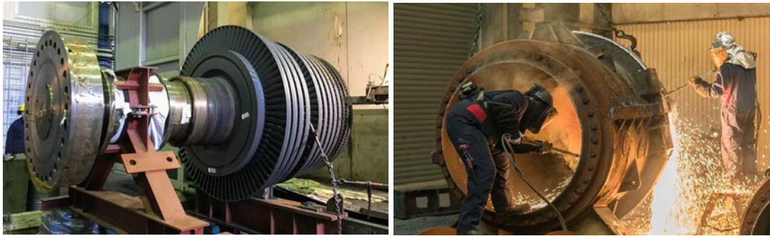
FIG. 6. Cold and thermal cutting operations.
