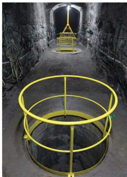
FIG. 2. Experimental deposition holes in the demonstration tunnel #2. Courtesy Posiva Oy.
