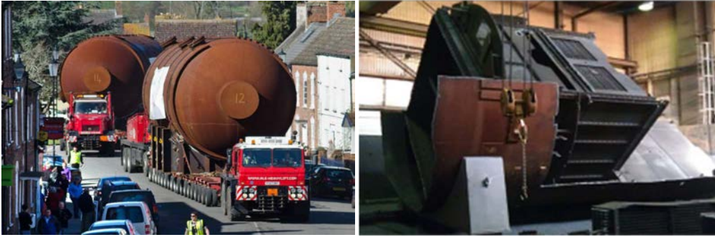
FIG. 9. Transport of Boilers (left) and partly segmented boiler (right).
