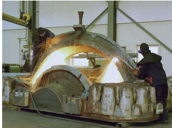
FIG. 13. NPP Würgassen turbine casing during segmentation at Cyclife site.
