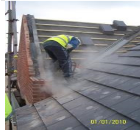
Poor Practice – Cutting roof tiles without control measures (National Federation of Roofing Contractors Ltd, GB)
