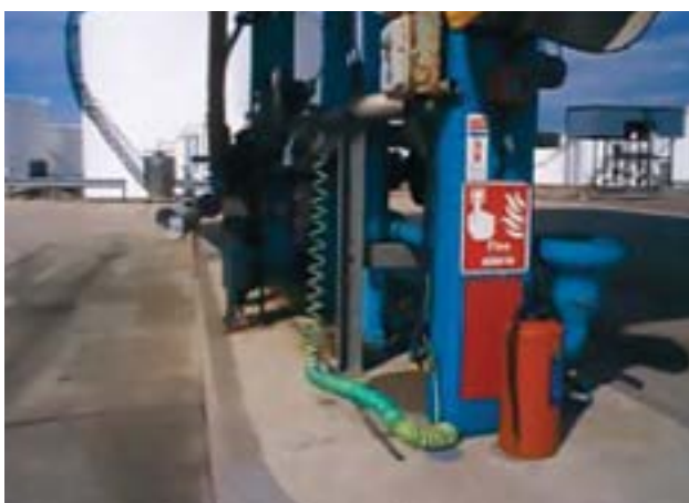
Figure 2. Typical bottom loading stand with provision for making earth connection to a tanker truck).
