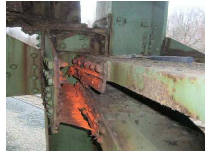
Fonte: BRIDGE INSPECTION MANUAL – NY'S DOT
