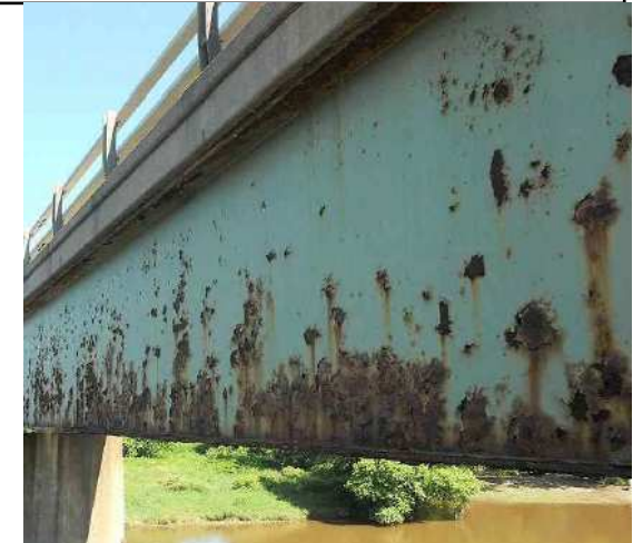
Fonte: BRIDGE INSPECTION MANUAL – NY'S DOT
