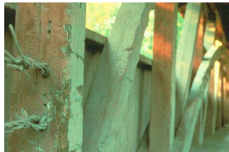
Fonte: BRIDGE INSPECTION MANUAL – NY'S DOT
