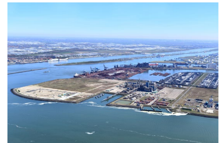
Port site Kop van de Beer, Port of Rotterdam. Photo Credit: Danny Cornelissen. Image courtesy of Port of Rotterdam Authority.
