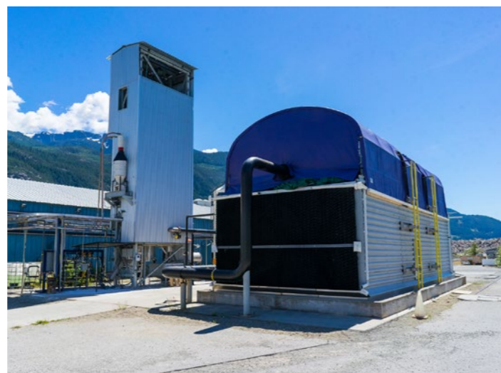
Carbon Engineering's pilot plant Direct Air Capture system. Shown are the air contactors and calciner (left). Image courtesy of Carbon Engineering Ltd.
