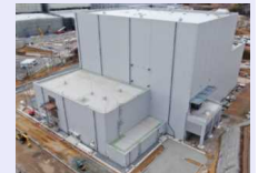
<Full view of the building>
