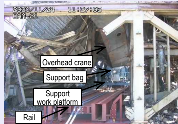
<Completed installation of supports for the overhead crane>
