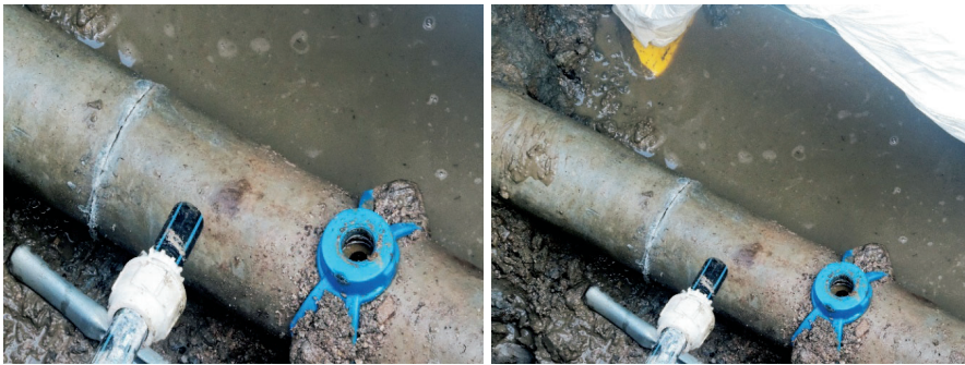
Figure 16 - Detail of the branch point.
