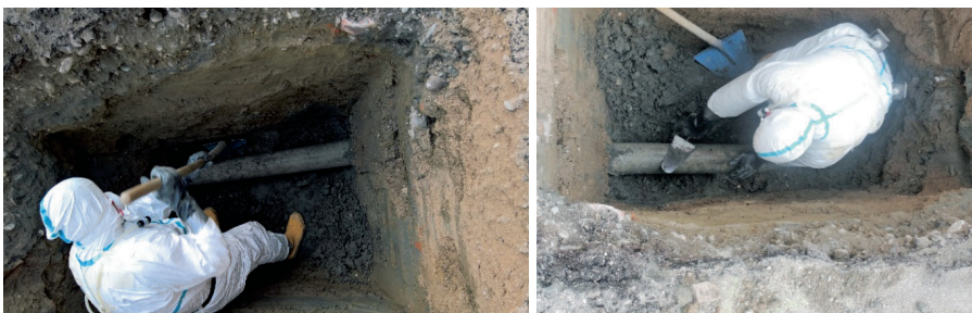
Figure 14 - Uncovering an asbestos-cement pipe using hand tools.
