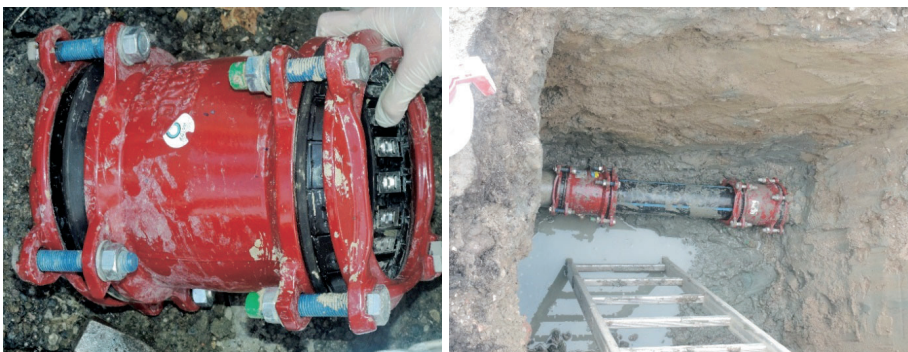
Figure 10 - Detail of the connecting joint (left); section of new pipe replacing the damaged pipe (right).
