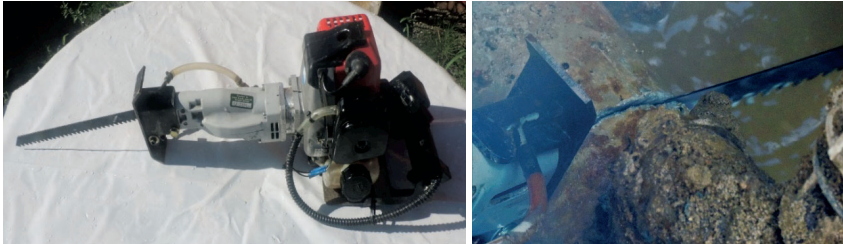
Figure 7 - Cutting a pipe with a low-speed petrol jigsaw.
