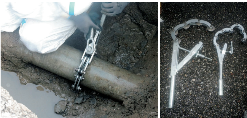
Figure 8 - Cutting a pipe with hand chain pipe cutters.
