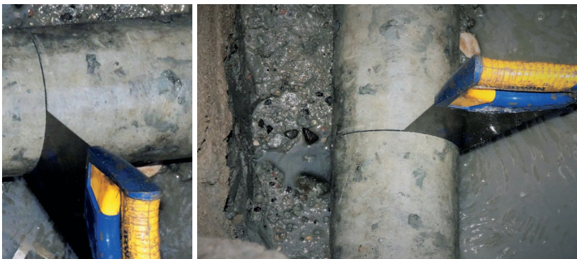
Figure 6 - Cutting a pipe with a hand saw (Inail Dit).
