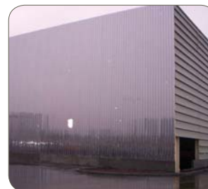
Tipo 1.4526/436, Ugine e Alz Steel Service Centre, Acelor Mittal Stainless, Katowice, Polonia
