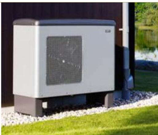
**Image 2.12:** Air source heat pump for space heating
