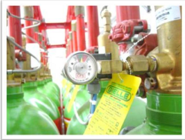
The search for halon 1301 replacements has been on-going for over 10 years and each alternative brings with it a unique set of properties. Gielle has brought to the market products that match the requirements of industry and latest research allows the company to introduce fire protection systems using Novec 1230 fluid, a new development with some advantages over current
