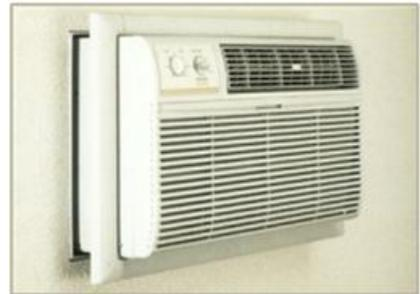
**Image 2.3:** Through-the-wall air-conditioning unit
