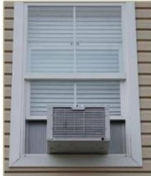
**Image 2.2:** Window mounted air conditioning unit
