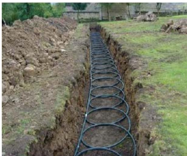
**Image 2.15:** Ground source pipework being installed
