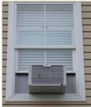
**Image 2.2:** Window mounted air conditioning unit
