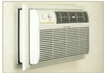
**Image 2.3:** Through-the-wall air conditioning unit
