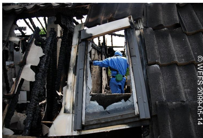
Asbestos removal work after a fire
