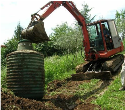
Figure 19. Vessel being dug out
