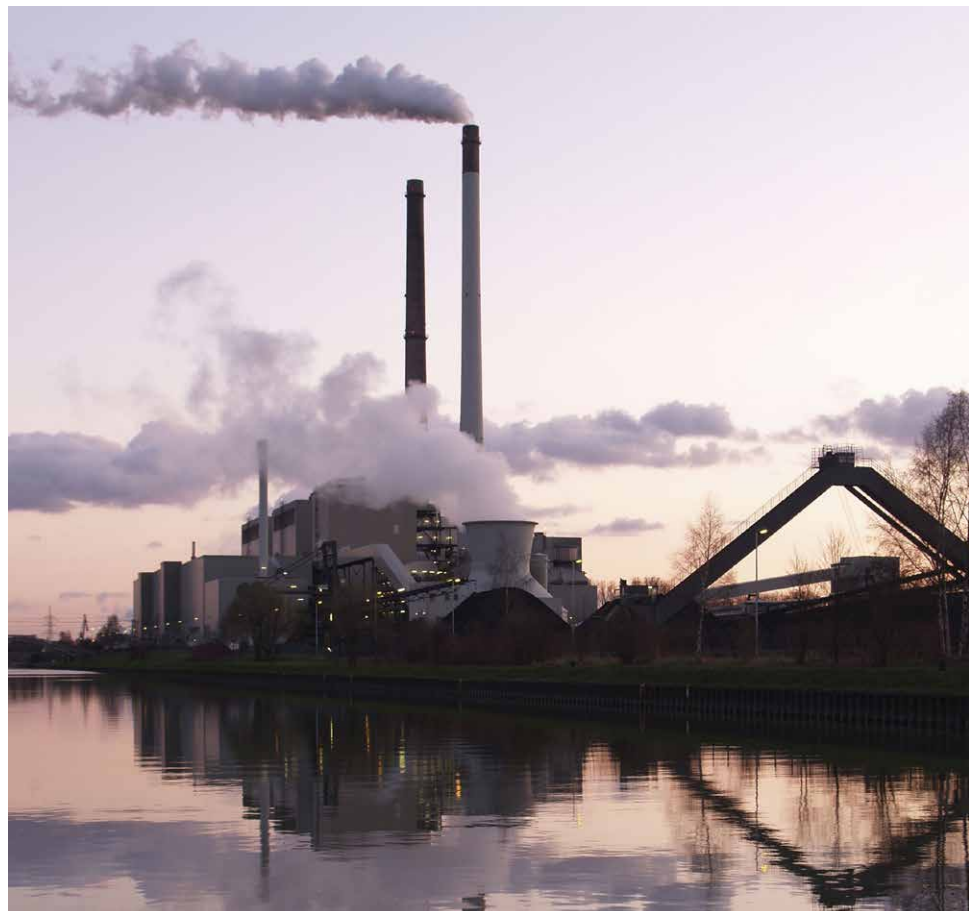
Coal power plant in Datteln (Germany) at the Dortmund-Ems-Kanal. Arnold Paul, 2006. Cropped by Gralo. Wikimedia Commons CC BY-SA 2.5 .
